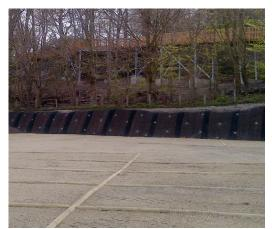
provide load bearing surfaces. The Cellweb<sup>®</sup> was positioned and infilled with the granular material and then topped with a decorative gravel.
